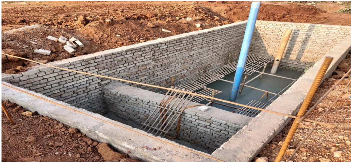
Fig. 2 Artificial Ground Water Recharging Pit under construction.
